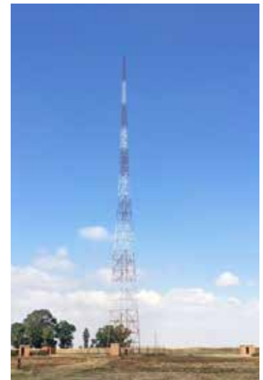
Picture: The existing mast, which is going to be decommissioned
